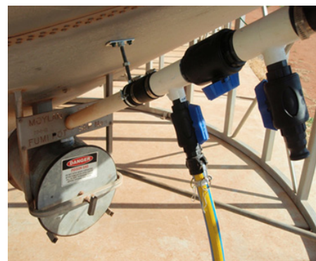
图 7 为了便于安装分接头系统, 我们切割并拆除了 550 mm 一段的管道 (40 mm)。考虑到分接头系统的额外重量, 安装了一个支架来支撑管道。使用两个 40 mm 橡胶套管连接 40 mm 管道。在橡胶套管上安装了四个软管夹, 并将其固定, 以完成气密安装。 Fig.7 A length (550 mm) of the 40 mm pipe was cut and removed to facilitate installation of the tap system. A brace was installed to support the pipe given the additional weight of the tap system. Two 40 mm rubber sleeves were used to connect onto the 40 mm pipe. Four hose clamps were installed to the rubber sleeves and fastened to complete the gas tight installation.
