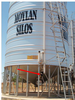
图 4 分接系统安装在现有的热虹吸管管道上。热虹吸管由 90 mm 雨水 PVC 管组成, 从筒仓顶部空间通向地面磷化氢应用室。磷化氢室具有进入筒仓底部的入口管道, 以完成再循环回路。 Fig.4 Tap system installed in existing thermosiphon pipework. Thermosiphon pipework consists of 90 mm stormwater PVC pipe leading from headspace of silo to ground level phosphine application chamber. Phosphine chamber has entry duct into base of silo, to complete the recirculation loop.
