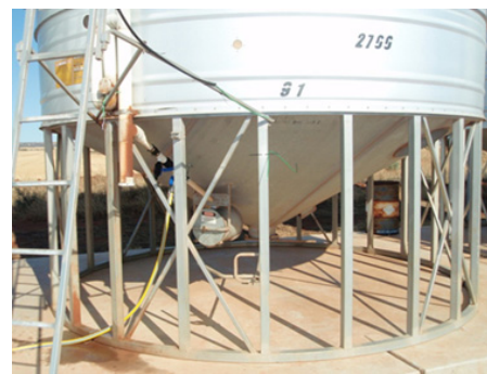
图 6 氮气通过分接头系统进入料仓, 该系统包含紫外线稳定球阀和凸轮锁接头, 便于软管连接。 Fig.6 Nitrogen is applied to the silo via tap system incorporating UV stable ball valves and camlock fittings for ease of hose connection.
