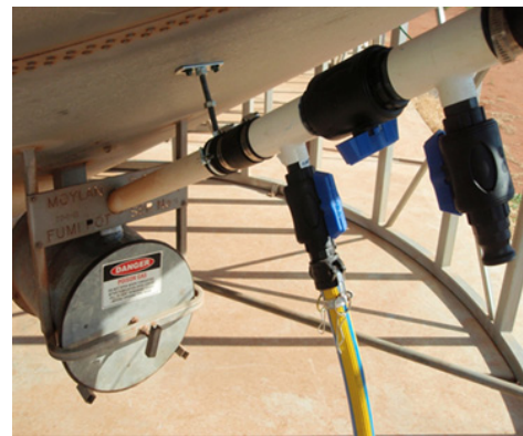
Fig.7 A length (550 mm) of the 40 mm pipe was cut and removed to facilitate installation of the tap system. A brace was installed to support the pipe given the additional weight of the tap system. Two 40 mm rubber sleeves were used to connect onto the 40 mm pipe. Four hose clamps were installed and fastened to complete the gas tight installation.
