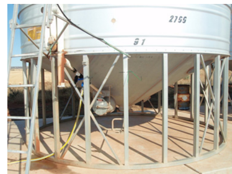
Fig.6 Nitrogen is applied to the silo via tap system incorporating UV stable ball valves and camlock fittings for ease of hose connection.
