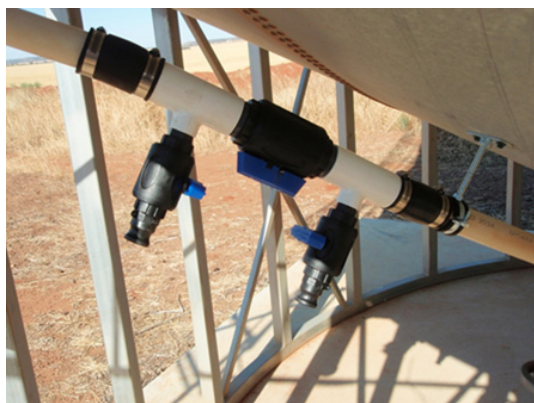
Fig.9 Once the Oxygen concentration in the Headspace and cone of the silo return values of 1% or less, indicating the presence of 99% Nitrogen, the Nitrogen production can be reduced and the exhaust ball valve closed. Briefly continuing a low flow (around 10 \text{ m}^3/\text{hour} ) of Nitrogen will build a slight positive pressure in the silo, which will aid in the silos ability to maintain high concentrations of Nitrogen. The N_2 application ball valve is then closed and hose withdrawn. The hose can be unfastened whilst still flowing Nitrogen as the flow is minimal. The inline ball valve is then opened allowing Nitrogen to circulate around the silo via the thermosiphon system, as dictated by the daily temperature fluctuations.
